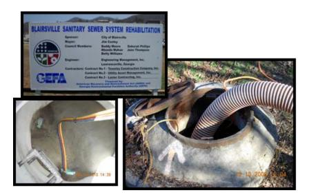
For many years the City of Blairsville experienced problems with inflow and infiltration of stormwater and groundwater leaking into the wastewater collection system. The City contracted with EMI to perform a Sewer System Evaluation that included a thorough analysis of the sewer system to identify all of the inflow sources.
